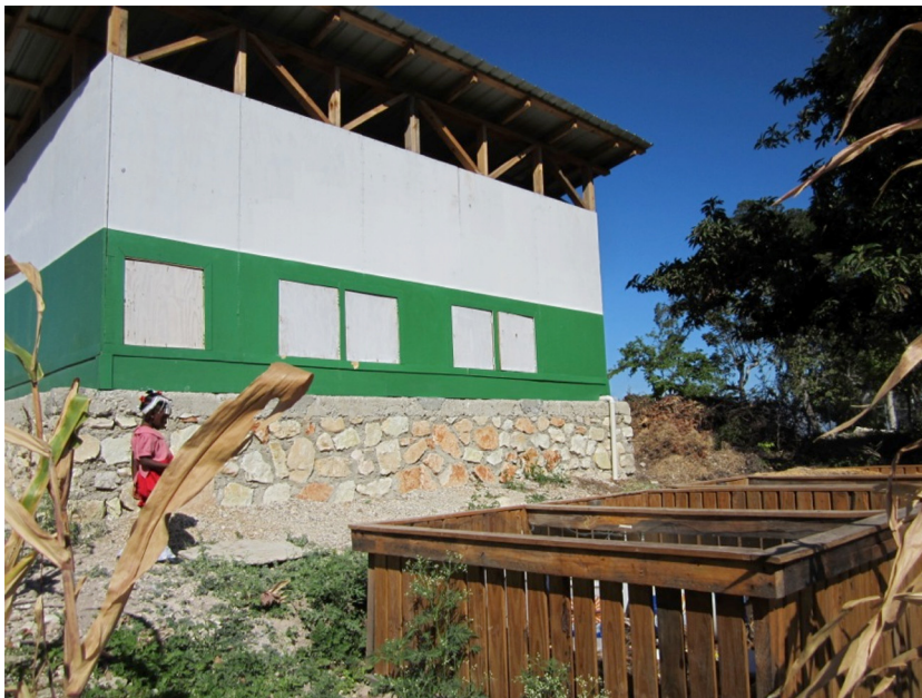
Fig. 12. Human waste composting latrines: designed by Give Love and maintained by local people, these latrines address a sanitation need, and the harvested compost is used in community gardens or sold.
