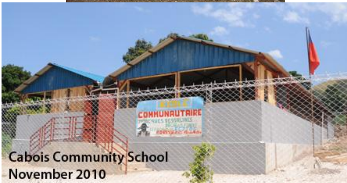
Cabois Community School Post-Earthquake
